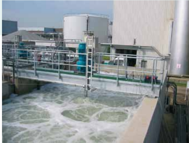
1 out of 9 HYPERCLASSIC®-Mixer/Aerators in an industrial wwp in Belgium (Pulp & Paper Industry)
