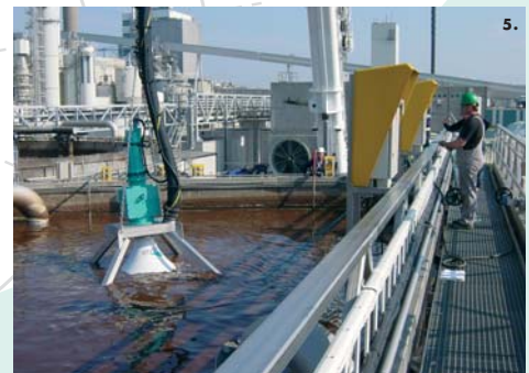
3.-5.: Installation of a HYPERDIVE® Mixing & Aeration System
