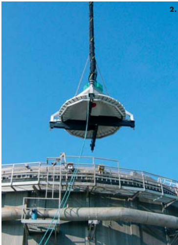
1.-2.: Installation of a HYPERDIVE® Mixing & Aeration System
