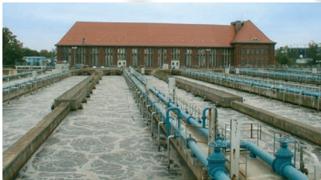
Installation of a TEX-FLEX aeration system in a municipal wastewater treatment plant in Germany
