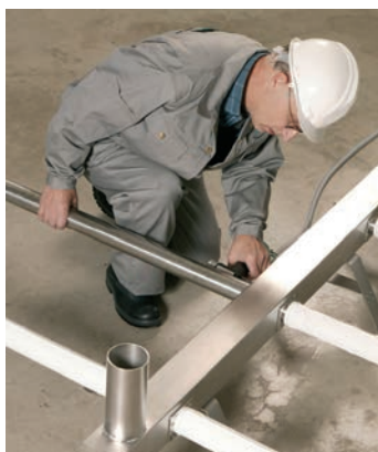
Installation of a TEX-FLEX aeration element
