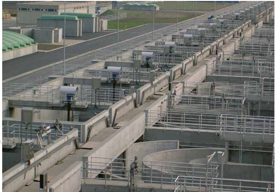
32 HYPERCLASSIC® -Mixers in the anaerobic basins in a large wwtp in Vienna, Austria
