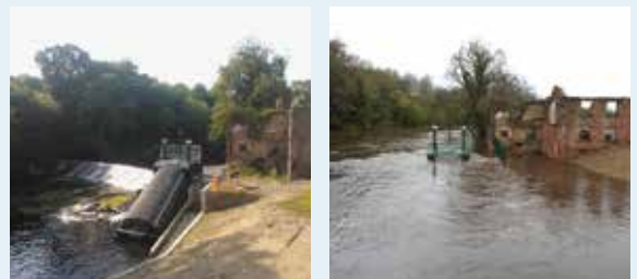
Before and after flooding at Goldsborough, UK
