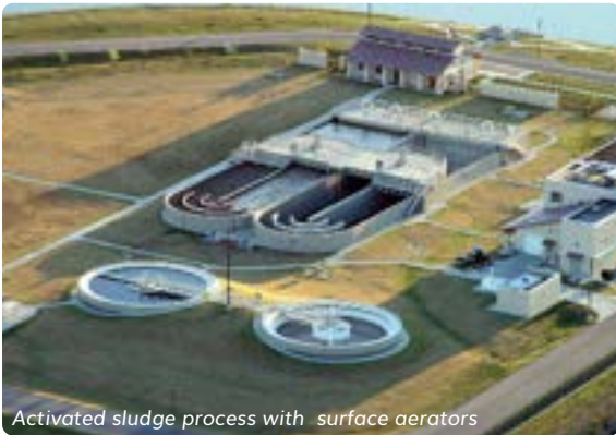
Activated sludge process with surface aerators
